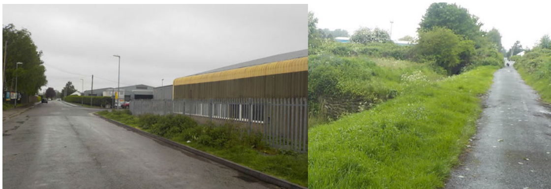
Figure 4 - Existing layouts at eastern end of New Bridge Lane (east)
