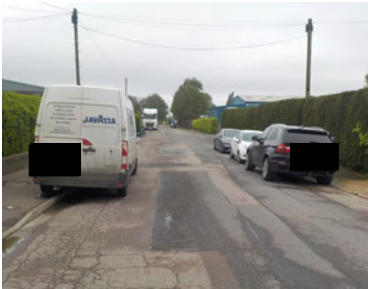
Figure 8 - Parking on New Bridge Lane
