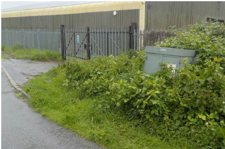
Figure 6 - Existing sub-station on New Bridge Lane
