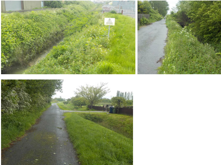
Figure 1 – Existing drainage features along New Bridge Lane (east)
